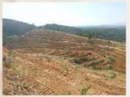
Completed terraces, roads & drainages
