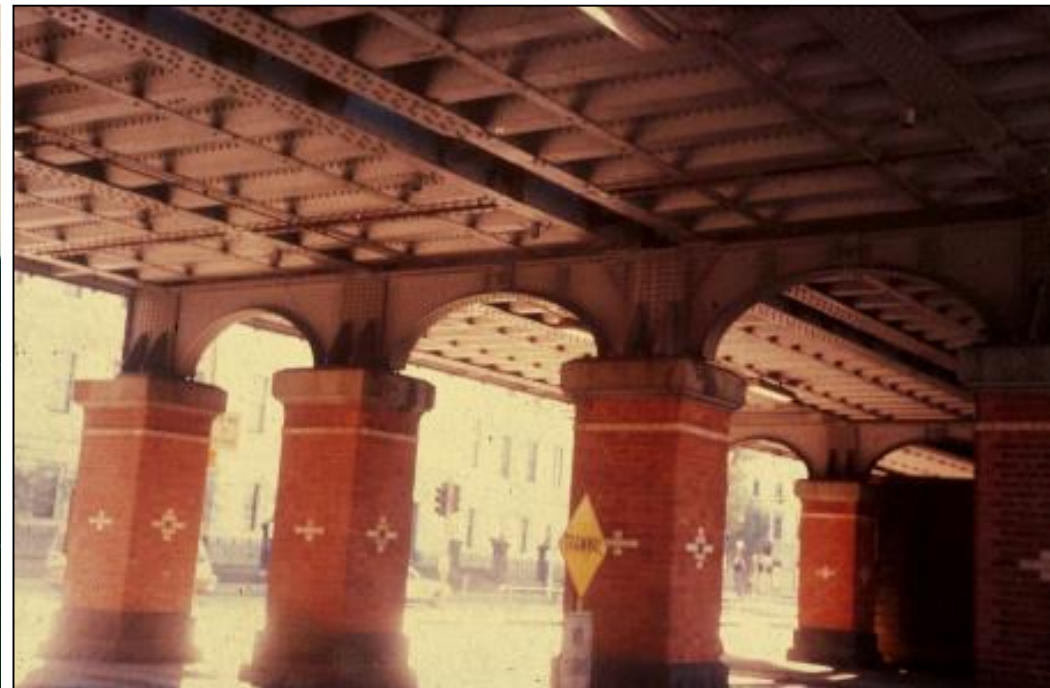
110-year old viaduct bridge in Melbourne Australia - still heavily trafficked structure
