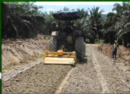
ROTOVATING TO THOROUGHLY MIX SOIL WITH PRE MIX CEMENT & CHEMICAL
